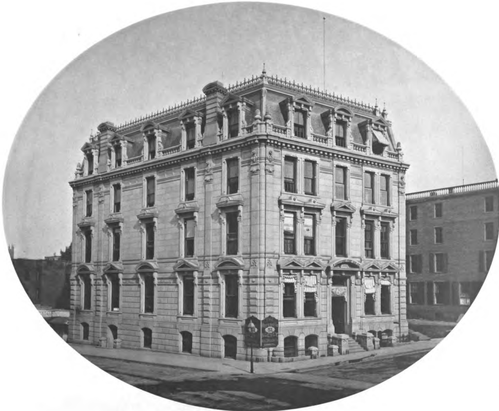
THE HARTFORD FIRE INSURANCE COMPANY'S BUILDING, ERECTED IN 1870.
