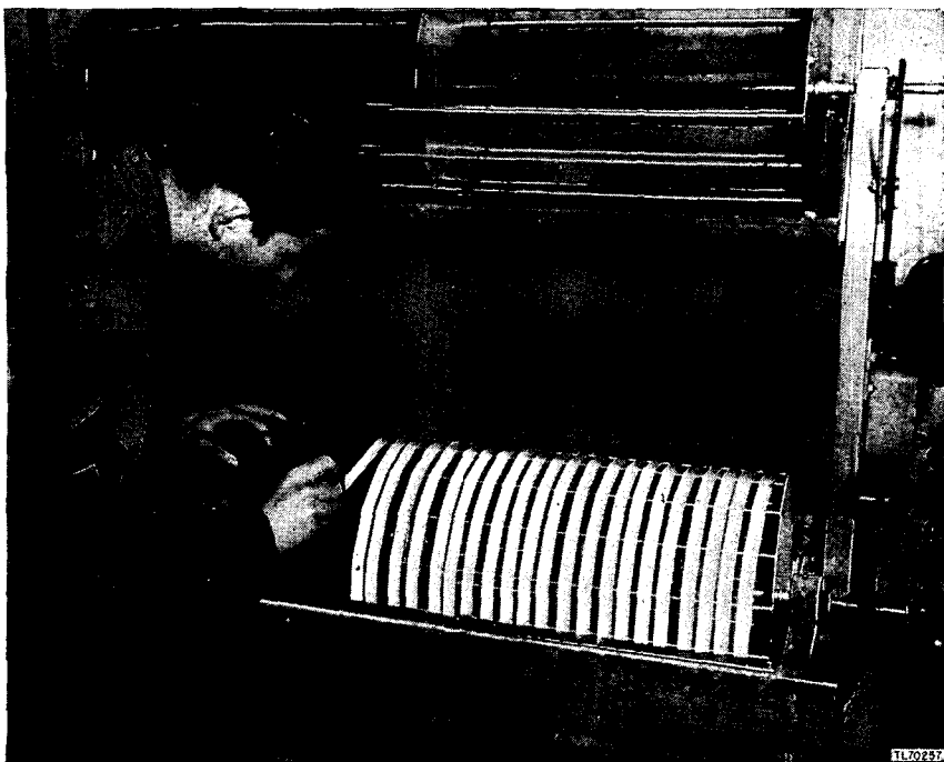
Figure 13. Loading film on reel for developing.
