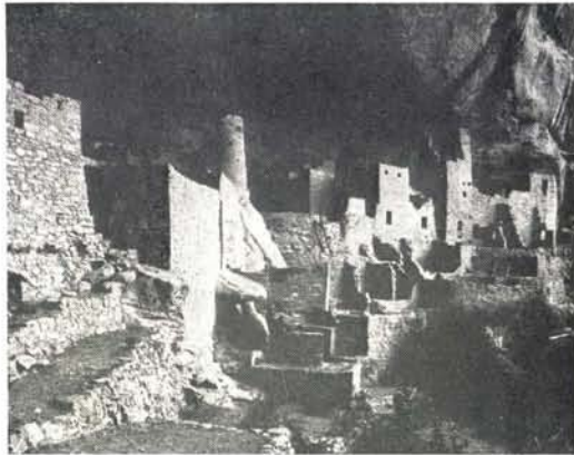
Cliff Palace, looking east—Mesa Verde National Park.
